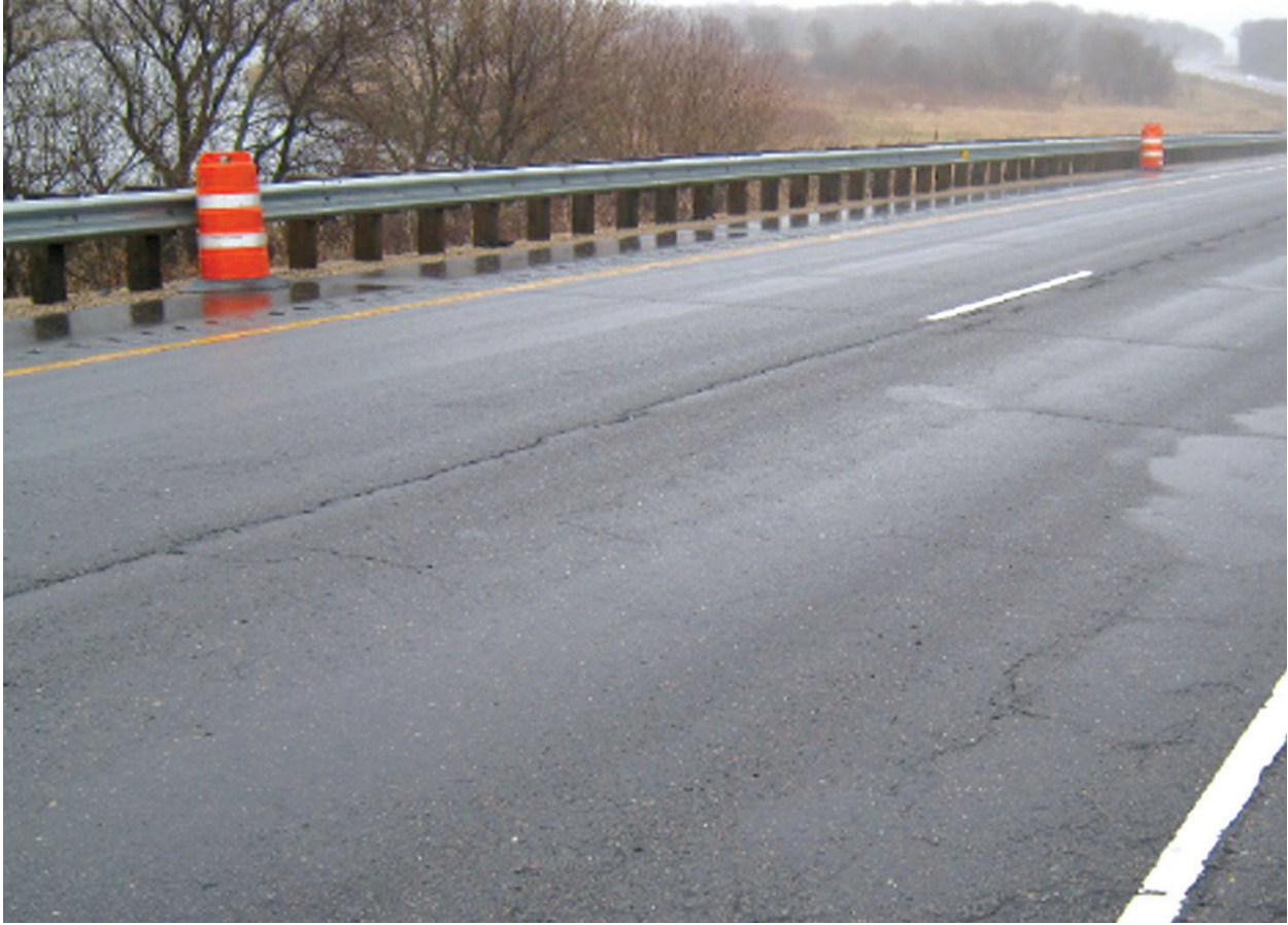
Figure 1. Example Block Cracking From Age-Related Embrittlement in Two-Year Old Surface
